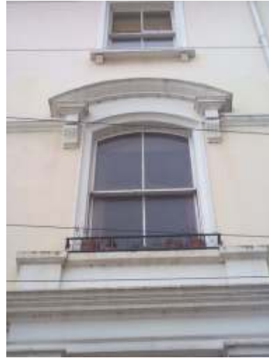
A 4 paned sash window typical of Clytha Square - Note hornless meeting rail
