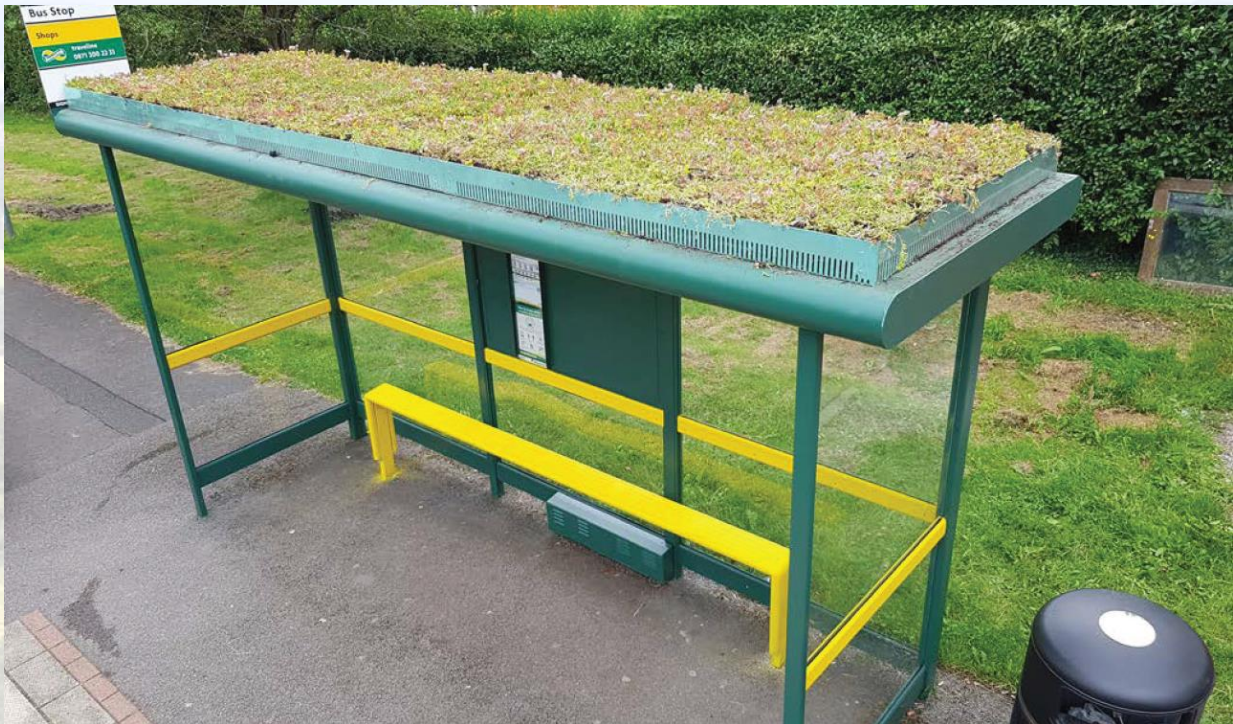
Retrospectively fitted and refurbished green roof shelter
