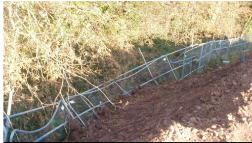
Heras fencing hasn't been secured and has been pushed over by the adjacent soil - this is not acceptable.
