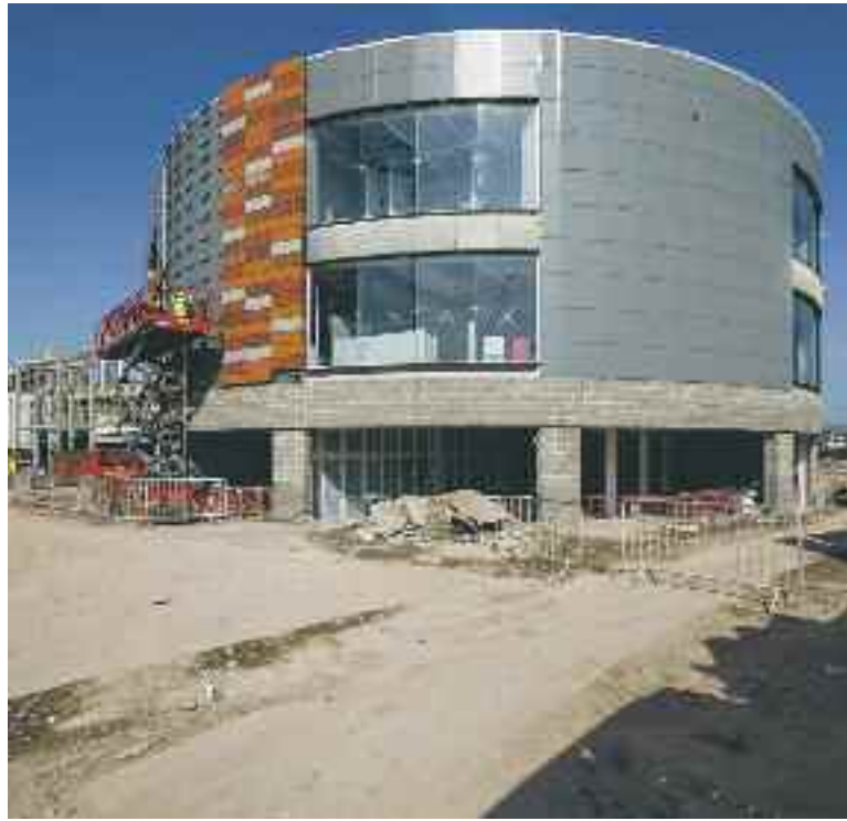
One of the new stores under construction
